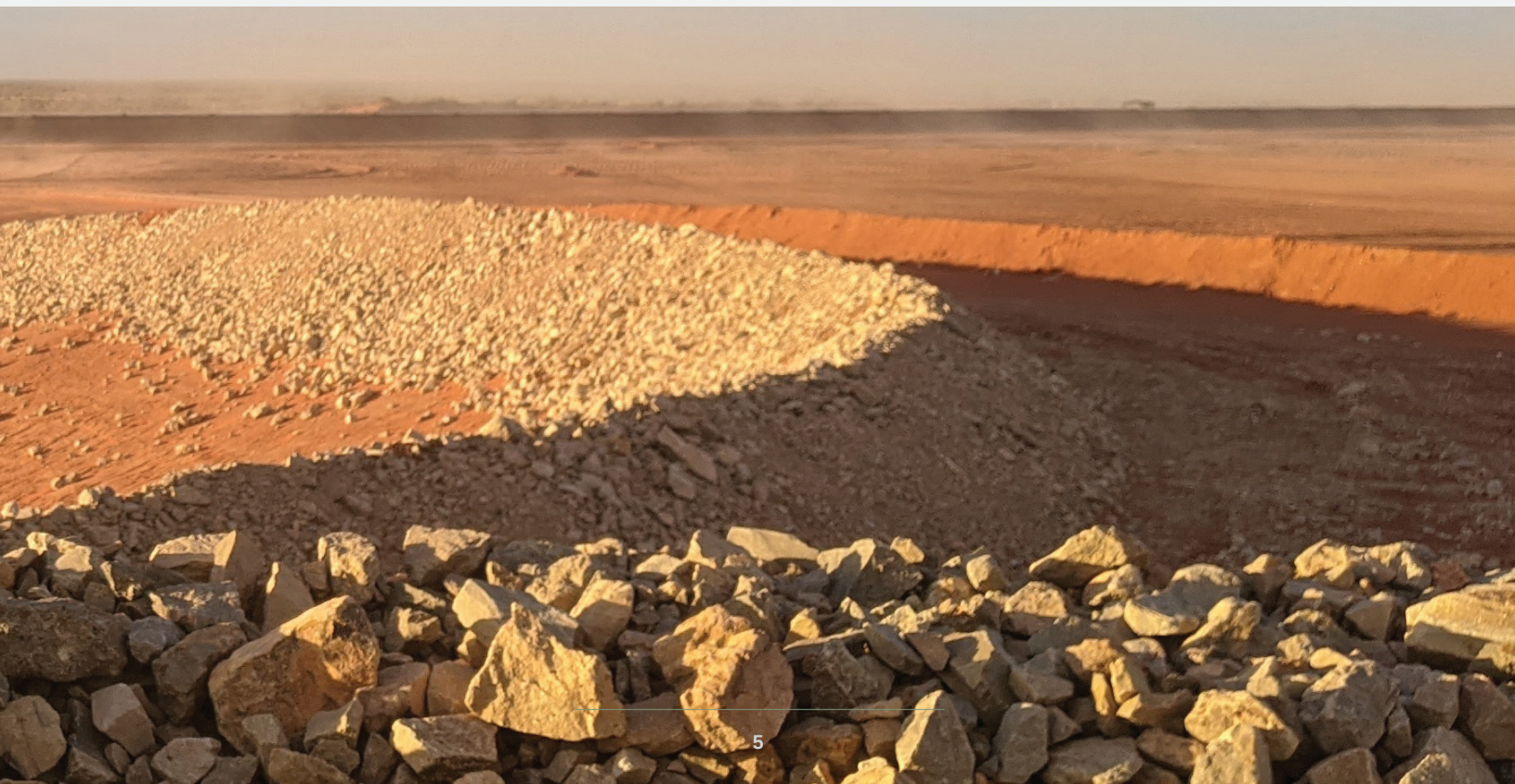
IMAGE: A COMBINATION OF DATASETS ON A TAILINGS DAM WALL CONFIRMING THE HEALTH OF THE UPSTREAM RAISES. GBG COMPLETED A SURFACE DTM COMBINED WITH A GEOPHYSICAL SEISMIC AND RESISTIVITY MODEL, WHICH WERE PHYSICALLY CALIBRATED WITH DRILL HOLES AND HYDROGEOLOGICAL MODELS. ALL DATA WAS INPUT INTO A 3D MODEL AND SUBSEQUENTLY ANALYSED IN LEAPFROG.
